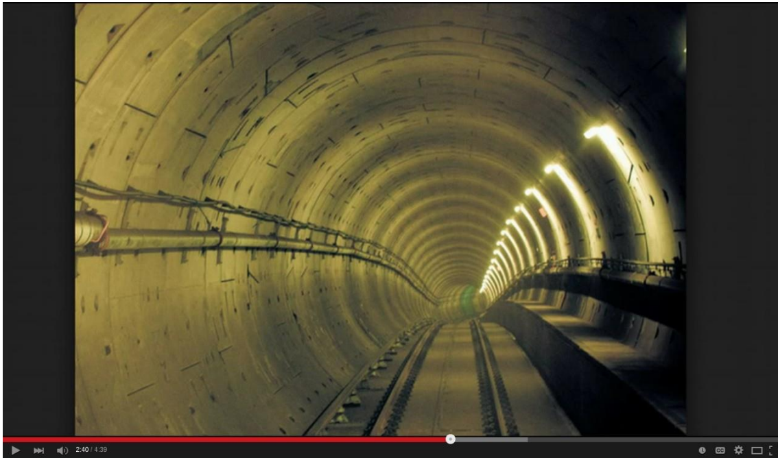
WALMART TUNNELS: DHS, NSA Venture Involves Hundreds of Stores
